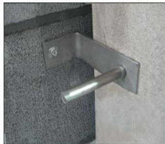
L Anchor w/Dowel - No Insulation
