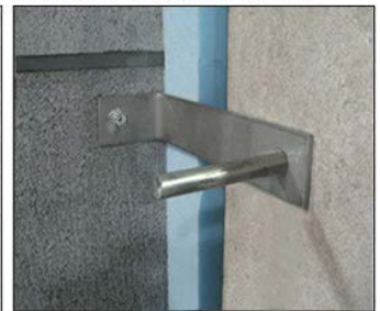
L Anchor w/Dowel with Insulation
