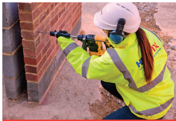
DryFix tie being power-driven into pilot hole
