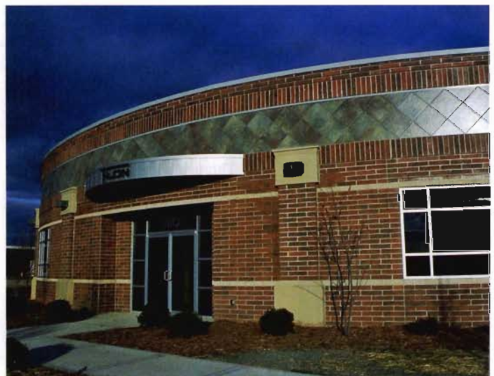
Single Wythe Half-High Construction in Hartland, Wisconsin
